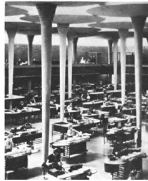
Johnson Wax Company offices, Racine, Wis., 1936, by Frank Lloyd Wright; interior of typing pool.
