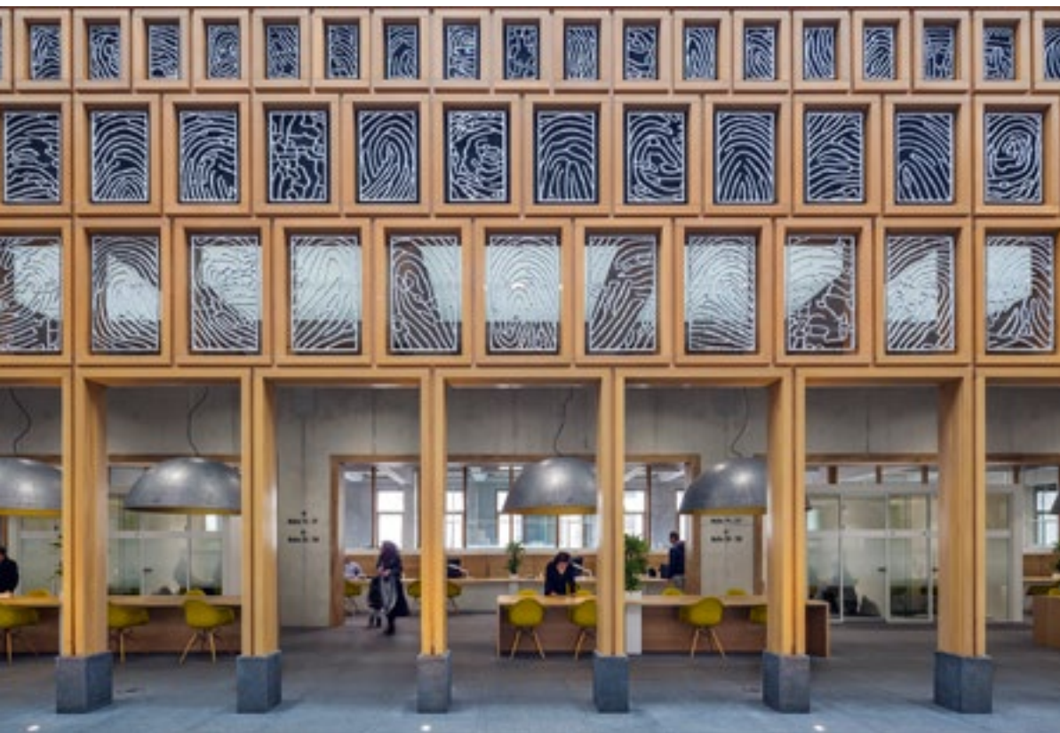
In the city hall in Deventer, the columns disappear in the uniform façade detailing. / In het Deventer stadshuis verdwijnen de kolommen in de uniforme geveldetailering
