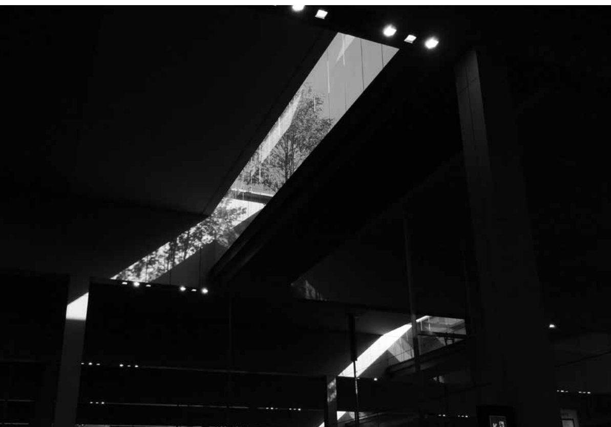
Koen van Velsen architecten, Public Transport Terminal Breda / OV-Terminal Breda, platform hall / perronhal
