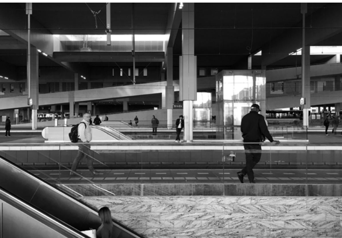
Koen van Velsen architecten, Public Transport Terminal Breda / OV-Terminal Breda, platform hall / perronhal
