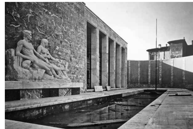
South side of the Palazzina Reale with exedra/ Zuidgevel van de Palazzina Reale met exedra
