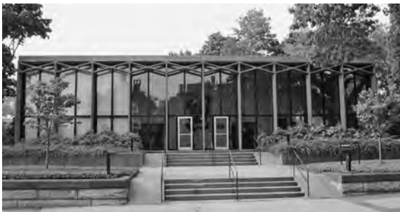
Philip Johnson, Computing Laboratory Building, Providence, RI (1958-1961)
