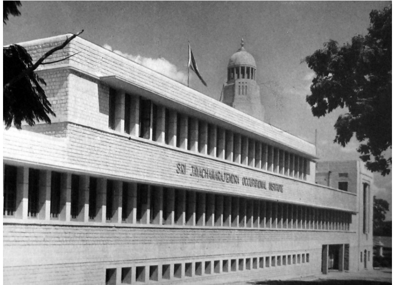
Use of local granite at the Sri Jayachamarajendra Occupational Institute, Bangalore, 1944 / Toepassing van lokaal graniet in het Sri Jayachamarajendra Occupational Institute, Bangalore, 1944
