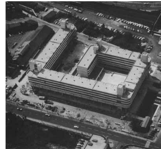
Lyons Israel Ellis, Southampton Central Area Development; Hampshire, 1969 Lyons Israel Ellis, Southampton Central Area Development; Hampshire, 1969
