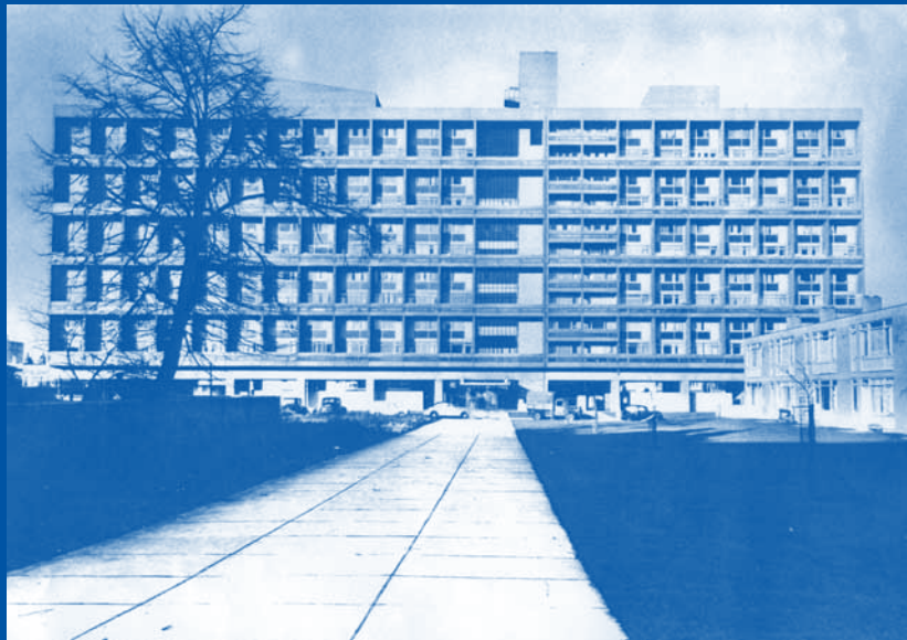
Hartlake Road. Extérieur / Exterior view
