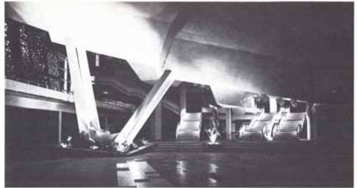
The main hall, Philharmonic building, Berlin
