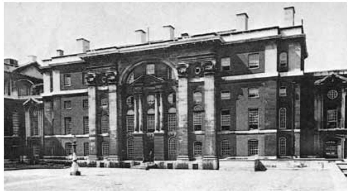
Greenwich Hospital, King William Block, Ostgevel/East façade
