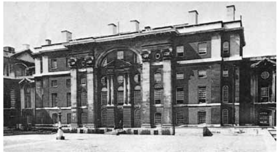
Greenwich Hospital, King William Block, East facade
