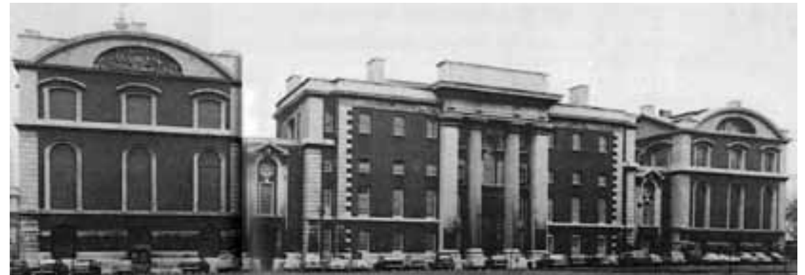
Greenwich Hospital, King William Block, West facade
