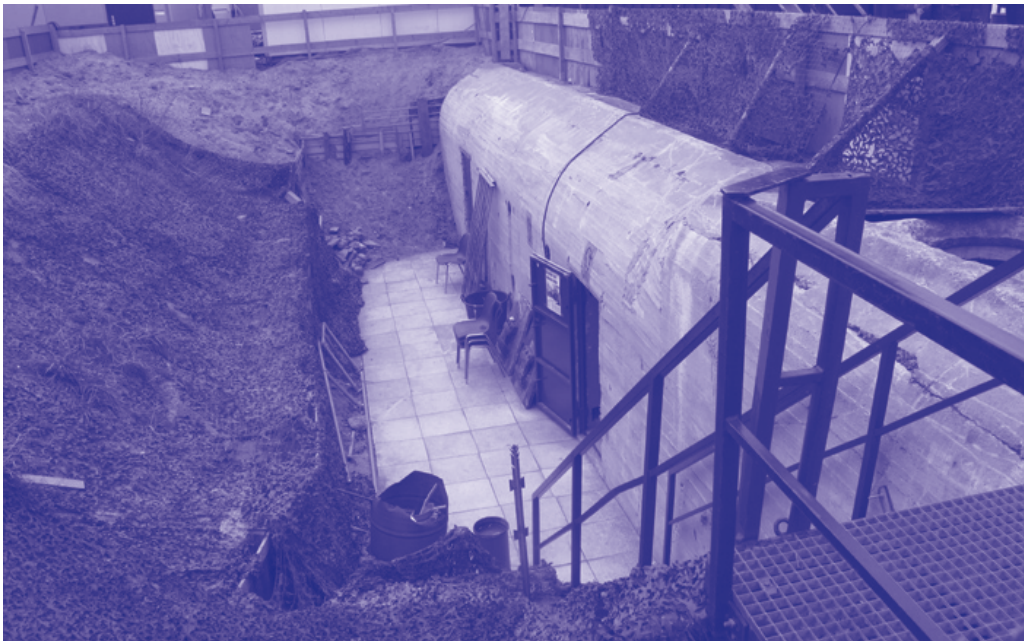
The excavated bunker on the Free Architecture Terrain in Scheveningen
