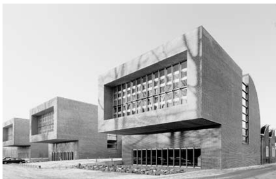
A-factory in Amsterdam, design / ontwerp: Neutelings Riedijk Architects, photography / fotografie: Jeroen Musch
