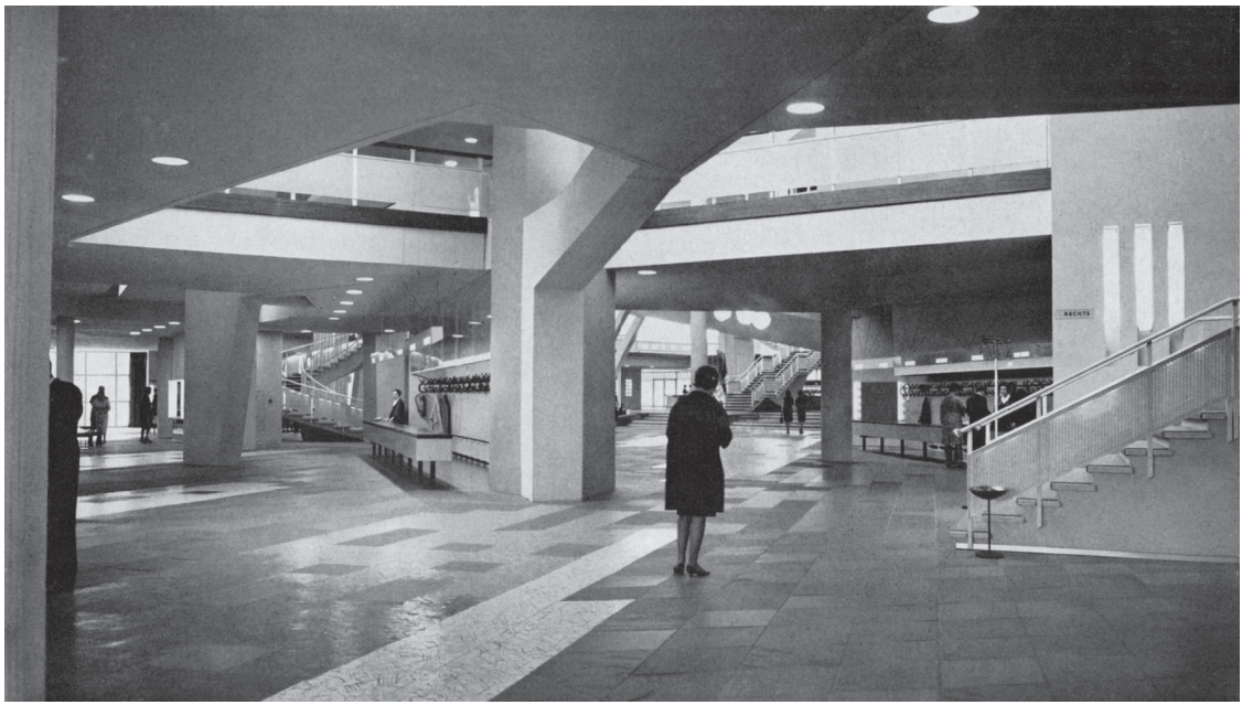
Lobby op begane grond / The lobby space at ground level
